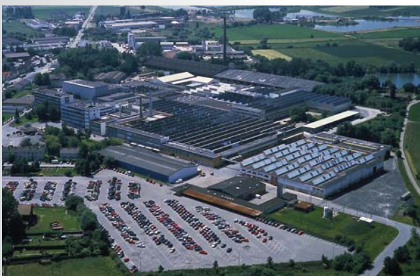
Stiebel Eltron's plant in Holzminden, Germany
